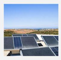
Source Hydropanels have been installed and demonstrated effective in 10 countries with highly variable climates, some with humidities as low as 10%.
